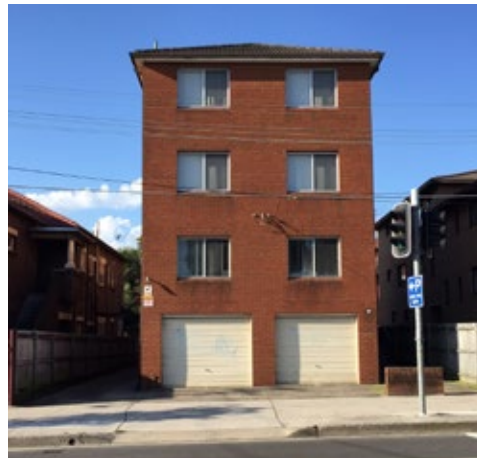
View of existing building at 16 Rainbow Street from Rainbow Street, Kingsford
