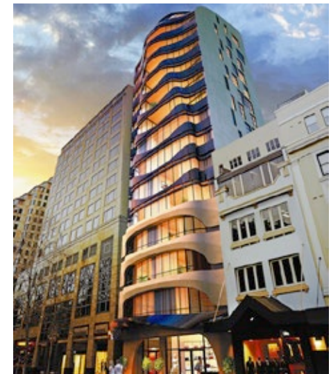
Figure 50: ‘Eliza’ 17 storey building, Elizabeth Street, Sydney Source: www.theurbandevolver.com
