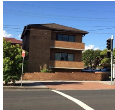
View of existing building at 18 Rainbow Street from Rainbow Street, Kingsford
