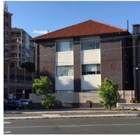
View of existing building at 63 Harbourne Road from Rainbow Street, Kingsford
