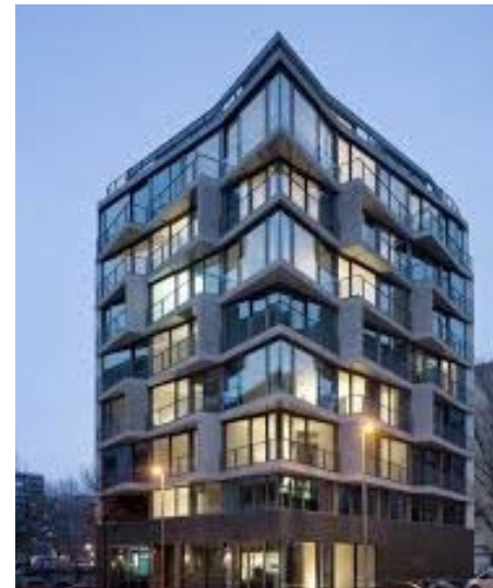
Figure 48: Nine storey apartment building, Berlin Source: www.sustainablecitiescollective.com
