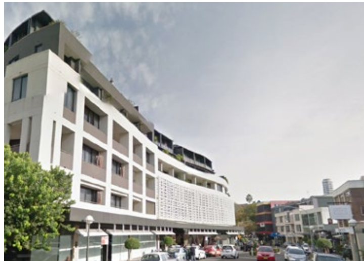
Figure 61: Four storey street wall, Double Bay Sydney Source: Google Streetview 2016
